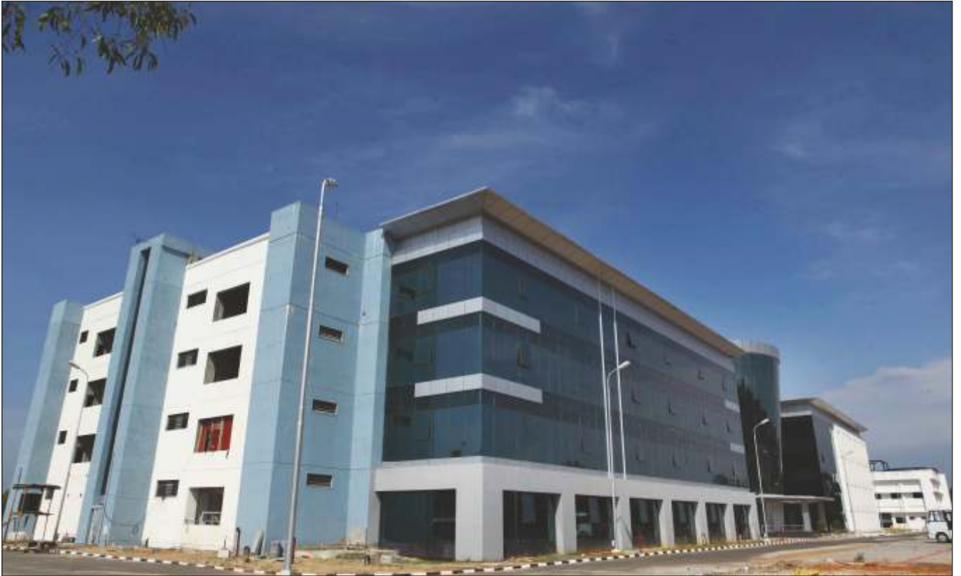
Chaithanya - SEZ building
