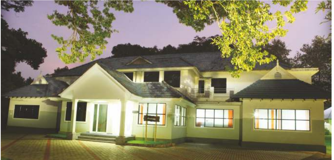
Villa Building - The traditional buildings renovated
