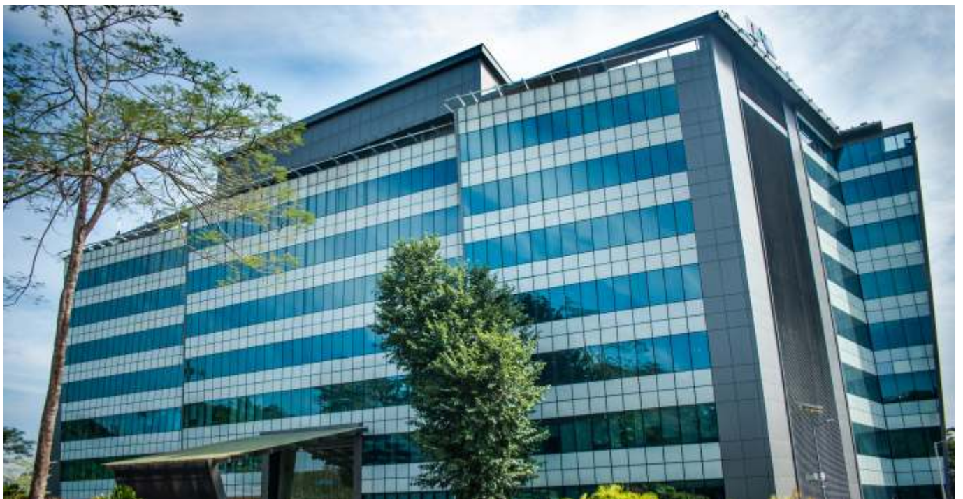
Indeevaram- SEZ Building
